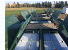
Secondary Treatment units
